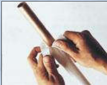
Fold back to reveal copper.
