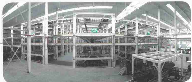
Threading, Air Pressure Test, and Anti-rust Treatment
