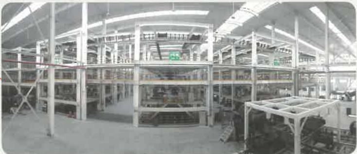
Threading, Air Pressure Test, and Anti-rust Treatment
